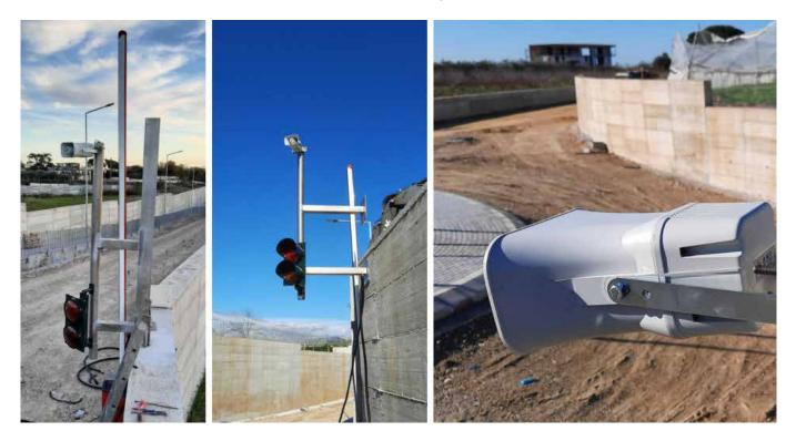
thus to be able to issue alerts when default critical thresholds are exceeded. Therefore, this **station** will **take care of activating traffic lights and sirens** connected to it on the basis of **alarm logics linked to the measurements observed both by the station on the Tusciano river and by the piezometric sensors directly connected to it**.
