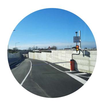
On behalf of GBL Costruzioni SUD srl, CAE installed a monitoring and early warning system for a new railway underpass in the Municipality of Battipaglia, which will be useful for inhibiting circulation in case of flooding, a situation that could occur during extreme flood events that are more and more frequent.
